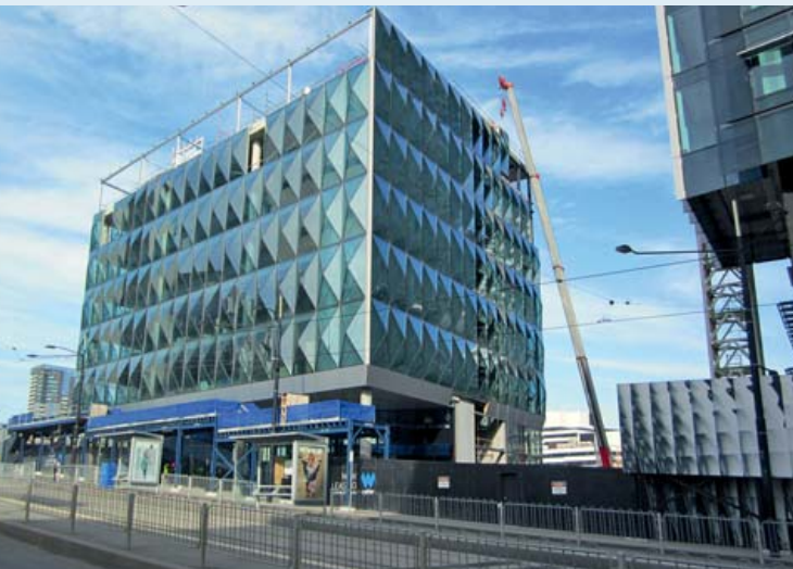
The Lantern Building in Collins Street, Melbourne is under construction.
