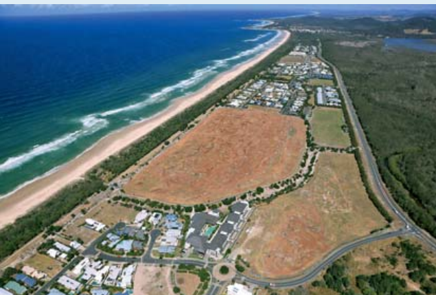
Aerial photograph of the site being prepared for the proposed Casuarina Town Centre.
