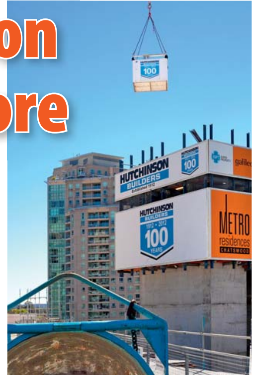
RIGHT: Hutchies on site at Chatswood in Sydney.
